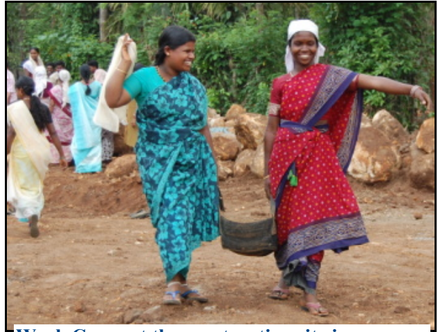
Work Camp at the construction site in progress
